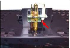
Undo the 4mm pipe with a 10mm spanner (see fig. 145) and disconnect from the pilot. Remove the bracket (see fig. 146).
