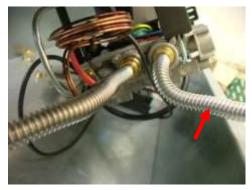
Supplied with the appliance is an isolation valve / pressure test combined (see fig. 90) fit this to the gas supply and connect the flexible inlet tube shown below (see fig. 91). IMPORTANT NOTE – Avoid kinks in the flexible gas pipe.
