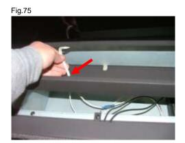
Undo the 4 screws at the back of the appliance to release the TTB (see fig. 76). Attach the two white right angled female connections to the TTB (see Fig. 77). Refit the access panel (Fig. 76).
