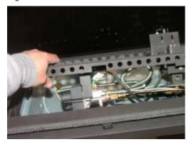
Disconnect the power lead, spark lead cable and 8 core cable from the controls box. (See fig. 32-35).
