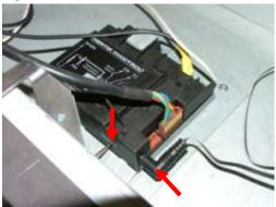
Bleed the gas through then attach the pressure test meter to the test point allowing length for the tube to travel through the appliance and out of the air intake (see fig. 99, 100)
