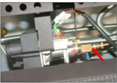
Only replace with genuine parts refitting in the reverse order. Test for soundness on all gas connection joints. Check Spillage.
