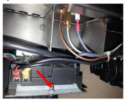
Remove the wiring from the controls black box. (see fig. 123)
