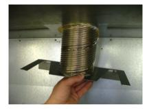
Push the spigot and liner back in place and secure the spigot via the 2 self tapping screws (see fig. 48). To ease the fitment of the inner casing the preferred gap between the spigot slide and top on the outer casing is 6mm (see fig. 49).
