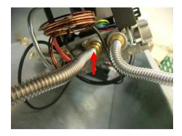
Supplied with the appliance is an isolation valve / pressure test combined (see fig. 57) fit this to the gas supply.
